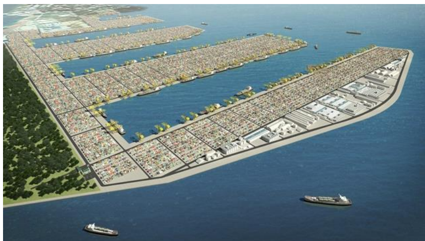
Tuas Mega Port project.
